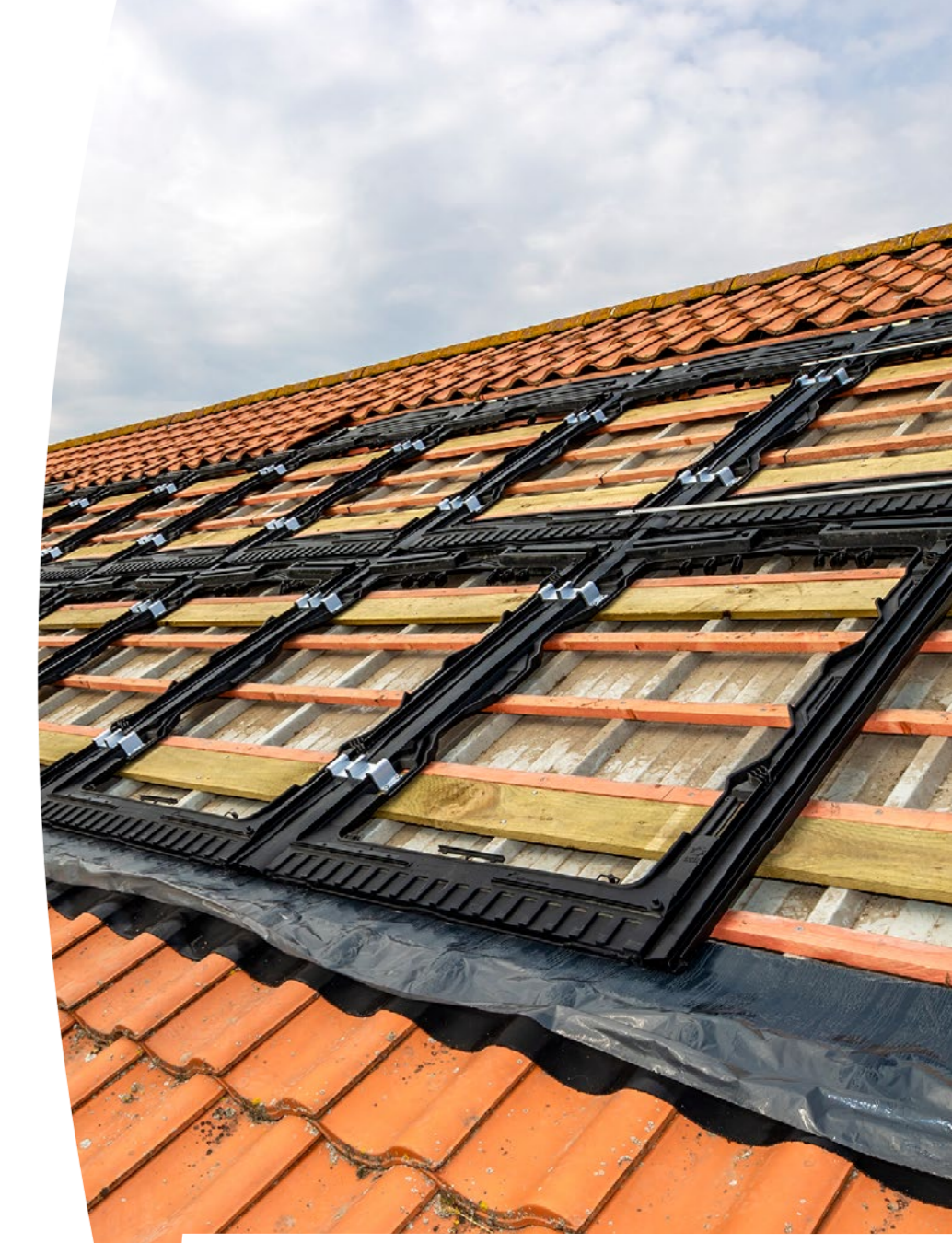
Solar panel installation, Hadleigh Country Park
